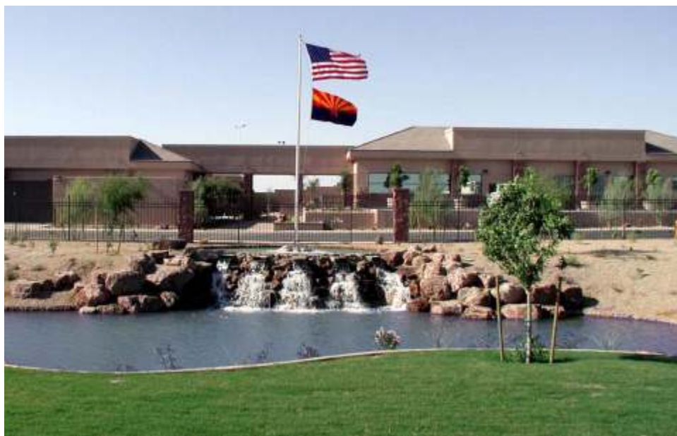
The aesthetically pleasing and environmentally friendly Palm Valley WRF is a welcome neighbor for several growing communities.
